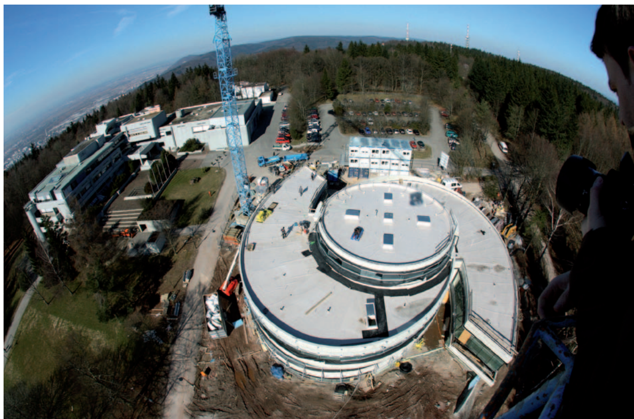
Fig. V.2.2a: Two neighbouring buildings: the main MPIA building and, still under construction, the HdA building. (2 March 2011)
