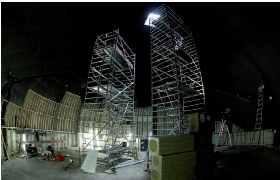
Fig. V.2.2d: Scaffolding in the Klaus Tschira auditorium in preparation for the installation of the planetarium dome (20 April 2011)
