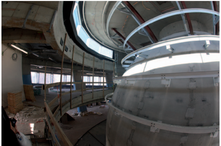
Fig. V.2.2c: Inside, the building's basic structure is now clearly defined. (22 March 2011)
