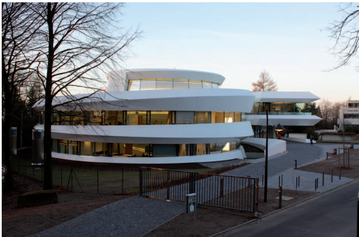
Fig. I.4.1: The HdA was finished in autumn 2011. The main entrance is to the right.
