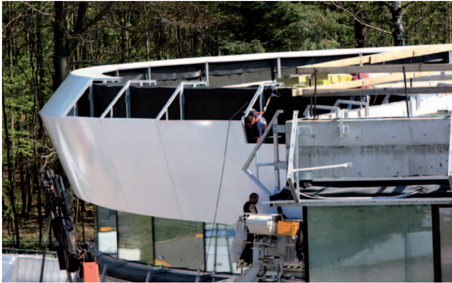
Fig. V.2.2b: Installing façade elements. (20 April 2011)
