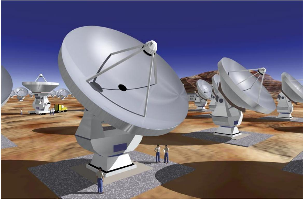
**Fig. III.4.10:** Artist's impression of Atacama Large Millimeter Array (ALMA). Up to 64 12 m antennas will be placed on the Chajnantor site, a high plateau at an altitude of about 5000 meters amongst the Andean mountains in Chile. (Courtesy of ESO)
