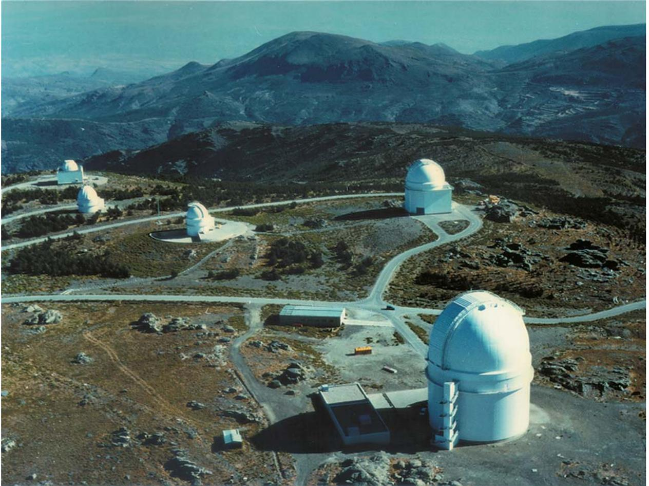
**Fig. I.2:** The domes of the telescopes on Calar Alto. From left to right: the Spanish 1.5 m telescope, the Schmidt telescope, the 1.23 m telescope, the 2.2 m telescope and the 3.5 m telescope.
