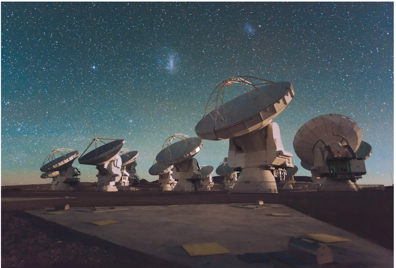
Fig. II.11.3: Antennas of the Atacama Large Millimeter/submillimeter Array (ALMA), a compound telescope on the Chajnantor Plateau in the Chilean Andes. The final ALMA configuration has 66 antennas acting like a single telescope.
