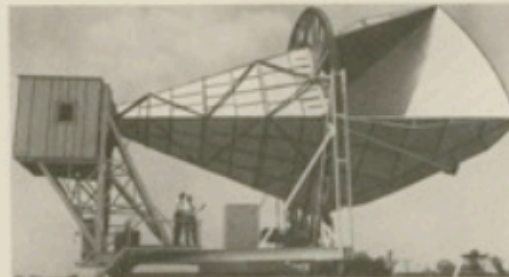
Giant ultra-sensitive horn-reflector antenna which received signals bounced off the satellite. It is located at Bell Telephone Laboratories, Holmdel, New Jersey.
